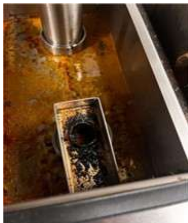
Photo 2 Sinks drain slowly and unit Overflowing into central section
