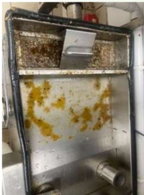
Photo 2 Sinks drain slowly and unit Overflowing into central section
